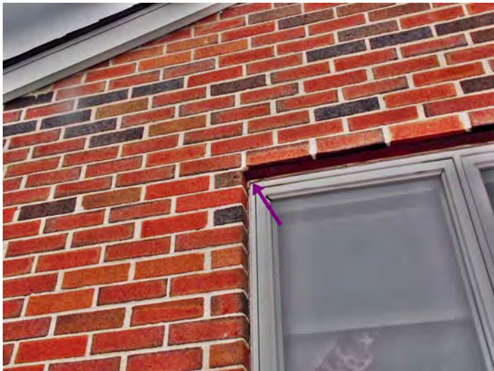
A window with cracked and dried caulking and a rusted lintel.
