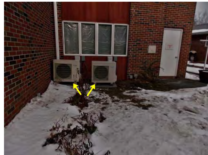
A pair of heat pump condensers.
