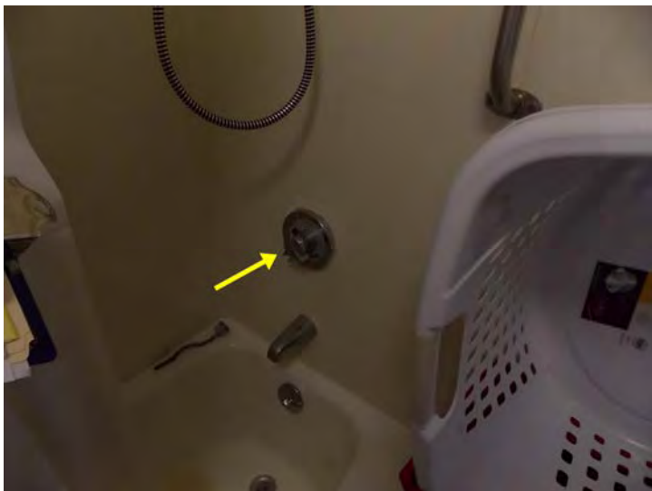
Bathtubs/showers have an anti-scald mixing valve.
