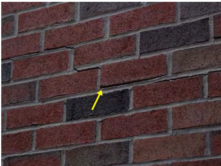
A close-up view of a step crack one the end section of a two-story building.
