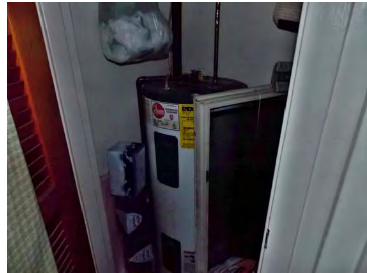
A typical apartment electric-heated DHW tank.
