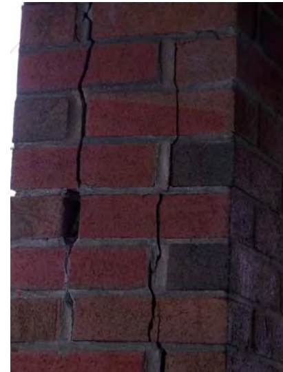
This arcade support column has cracks along the brick work.
