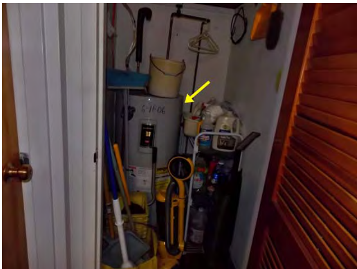
This is the electric-heated DHW tank that serves the community building.
