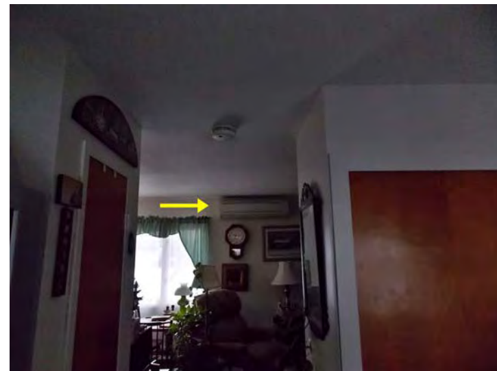
One of the heat pump terminal (blower) units in an apartment.
