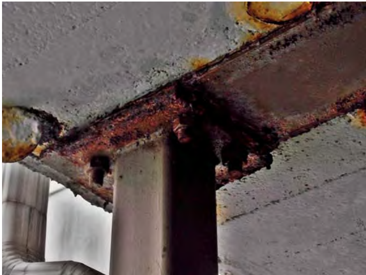
This arcade support has significant rust.
